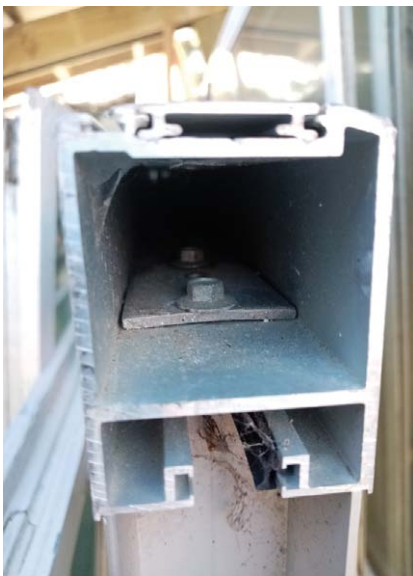
BOTTOM, LEFT - Not much insulation. Photo by Stephen Moller.
