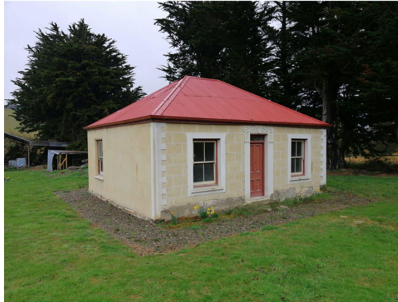
Gay Tans at Macraes – Rendered mud brick. An example of a bigger structure.
