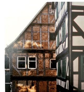
Straw-clay, plaster and timber in Germany
