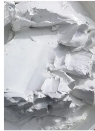
Lime putty ready to apply to walls
