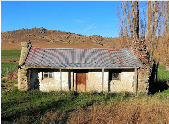
Murphy's Cottage in Fruitlands built in the 1870s approximately. Unattended Cob Building.
