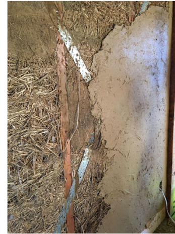
Clay plaster on the strawbale walls
