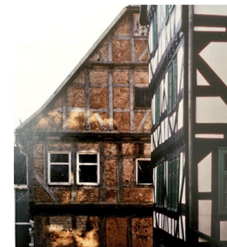
Straw-clay, plaster and timber in Germany
