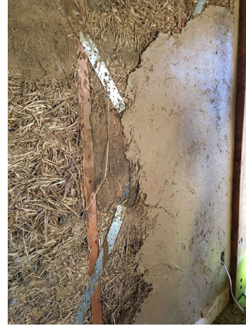
Clay plaster on the strawbale walls
