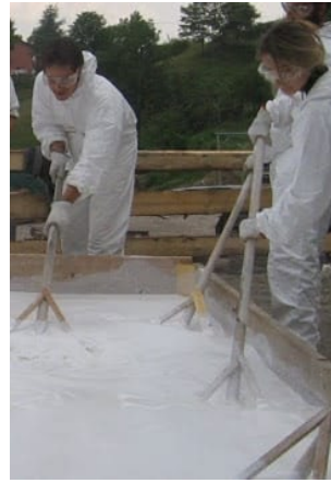
Hydrated lime mixed with some water
