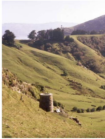
Traditional burning of the limestone to change the chemical properties
