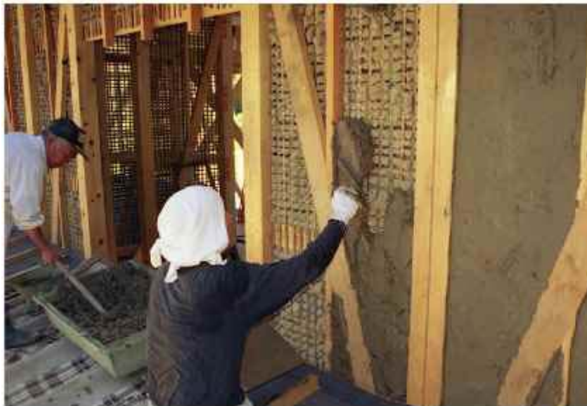
Fig. 11, Plastering Arakabe on bamboo lath
