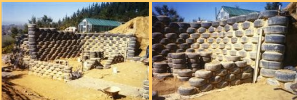
Construction of an Earthship, Hamilton area
